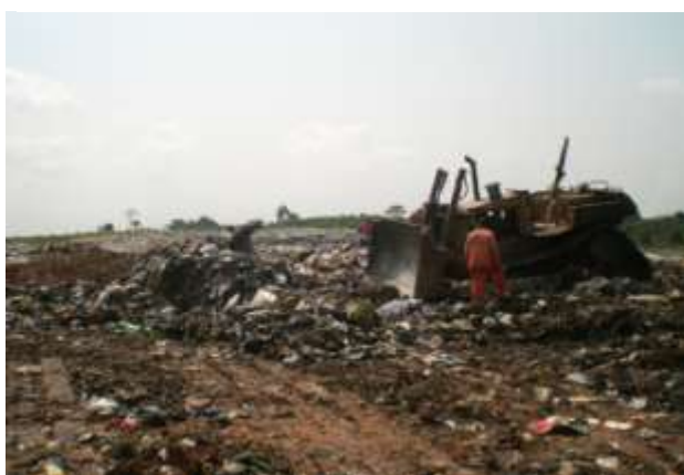
Up-hill view of the landfill with a compactor in site
