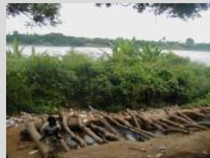
Plate 2: Latrine built with local materials without a superstructure close to the banks of Volta River
