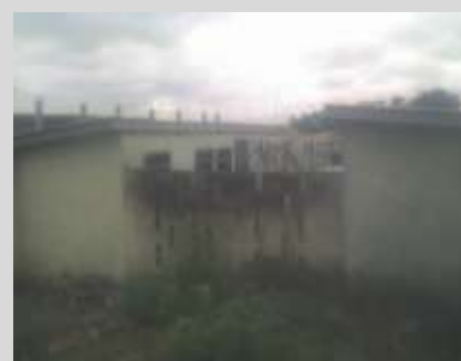
Plate 2: : Old dilapidated 12 seater KVIP.
