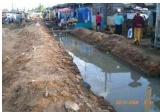
Plate 2: Excavation of trench for construction of drains. High water table posing as a challenge, Hide Link-Eastern.
