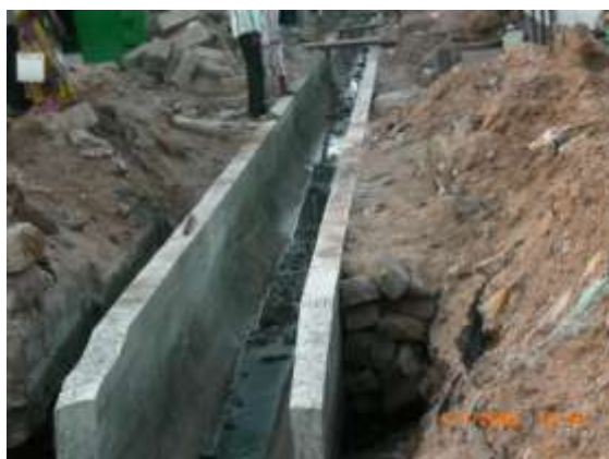
Plate 6: Constructed 750mm Ø drain which discharges into the roadside drain on the Oblogo street
