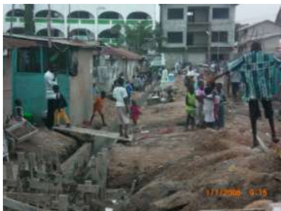
Plate 9: Drain cast on section of Western Side of Alhaji Street. Lamprey Mills Academy in the Background across Oblogo Street
