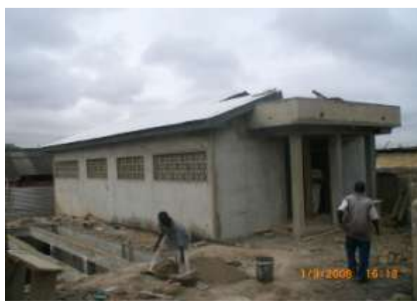
Plate 10: Superstructure roofed and rendered, ready for painting.
