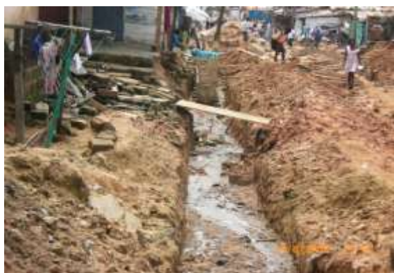
Plate 3: Excavation of trench for construction of drains, Hide Link-Western.
