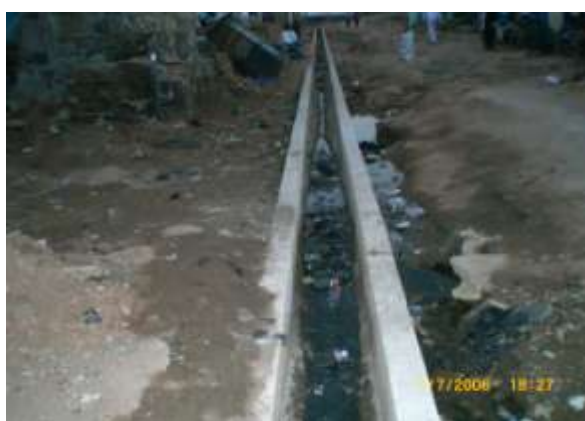
Plate 5: Constructed 450mm Ø on Eastern side of Hide link
