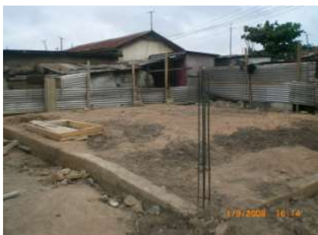
Plate 11: Foundation and blockwork for sides of refuse holding completed to receive hard core filling.
