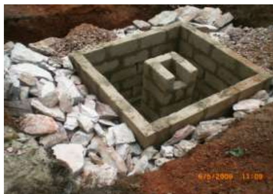
Plate 6: Soakaway for Holding tank under construction
