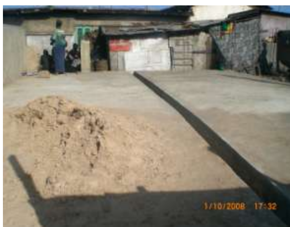
Plate 12: Floor slab of solid waste holding bay completed.
