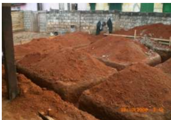
Plate 2: Excavation works for foundation of 1 No. 8-Seater WC Toilet for Laterbiokohie 2&3 Primary School
