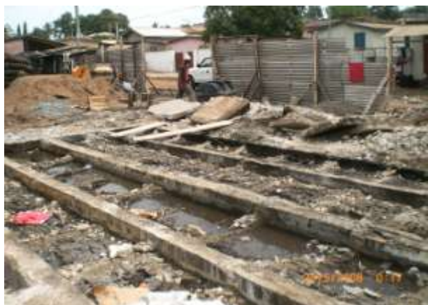
Plate 3: Existing holding tank for the old aqua privy ready for desludging
