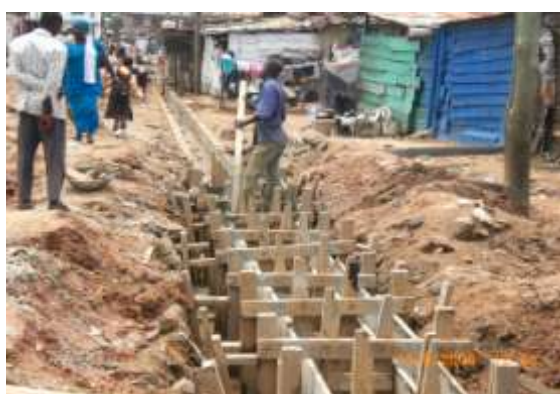
Plate 4: Formwork in place for pouring of concrete (foreground) and constructed concrete drain (background)
