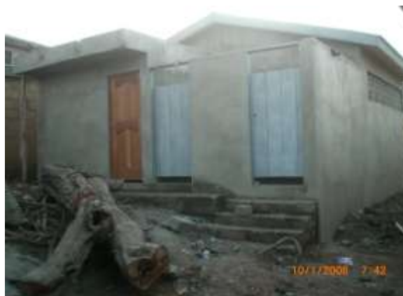
Plate 4: Superstructure for Da-Awatul Islamic Primary School completed. Ready for tiling and terrazzo floor finish. Roof slab provided to accommodate overhead water tank. Urinal facility designed to be opened to the elements of the weather
