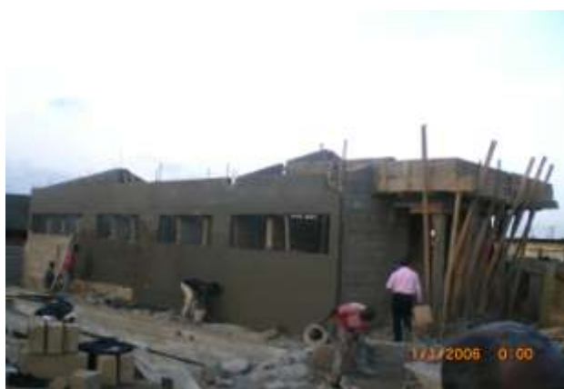
Plate 9: Works on 20 seater WC toilet facility at roof gable level.
