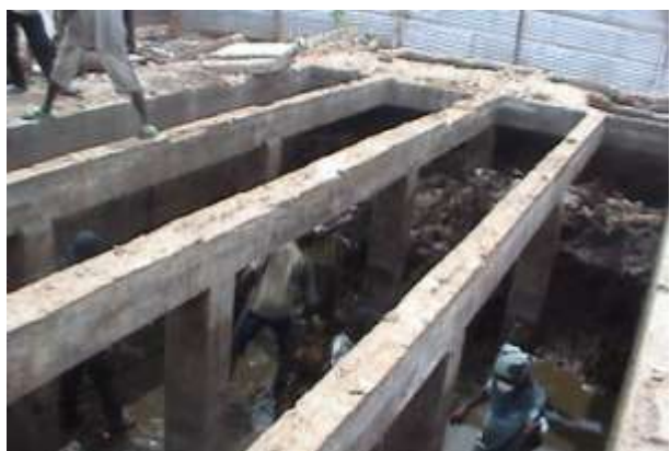
Plate 5: Holding tank of demolished aqua privy being desludged.
