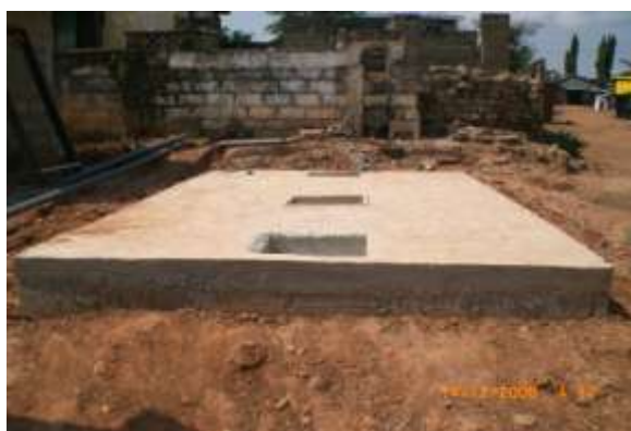
Plate 5: Roof slab of septic tank constructed
