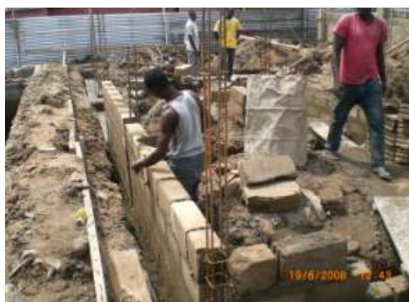
Plate 4: Foundation works for 20 seater WC toilet.
