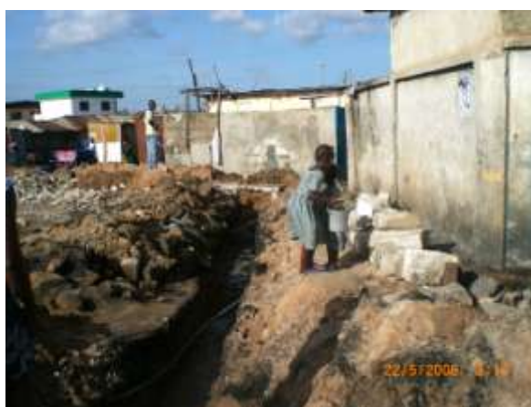
Plate 2: Excavated trench for the construction of fence wall
