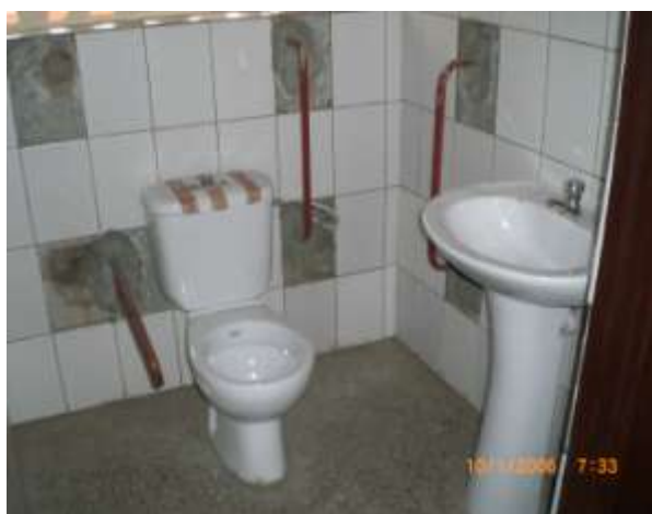
Plate 19: Cubicle for the physically challenged with metal bars fixed to provide support.
