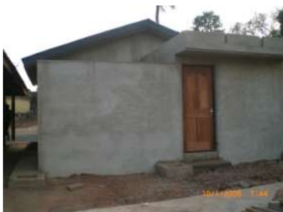
Plate 3: Superstructure for Laterbiokoshie 2&3 Primary School completed. Ready for tiling and terrazzo floor finish. Roof slab provided to accommodate overhead water tank. Urinal facility designed to be opened to the elements of the weather
