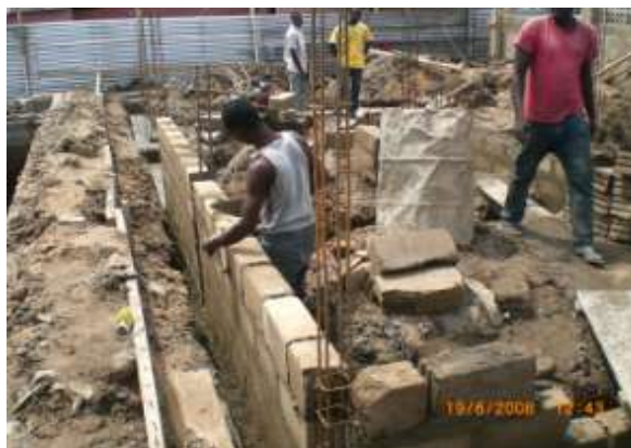
Plate 6: Sub structure of 20 seater WC toilet being constructed.
