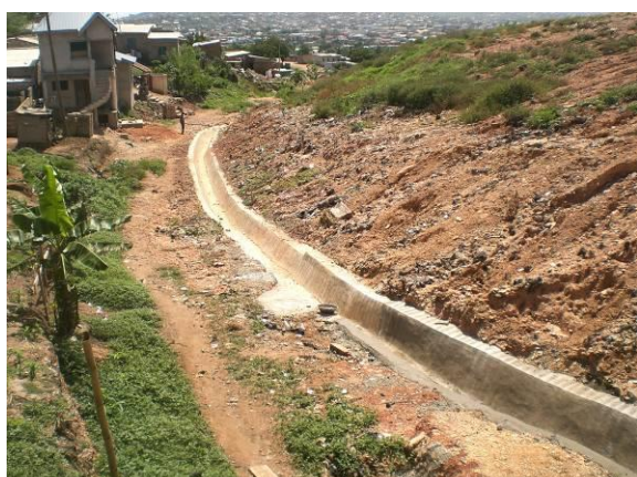
Plate 5: Peripheral drain for conveying surface run-offs from site into existing drainage systems in community
