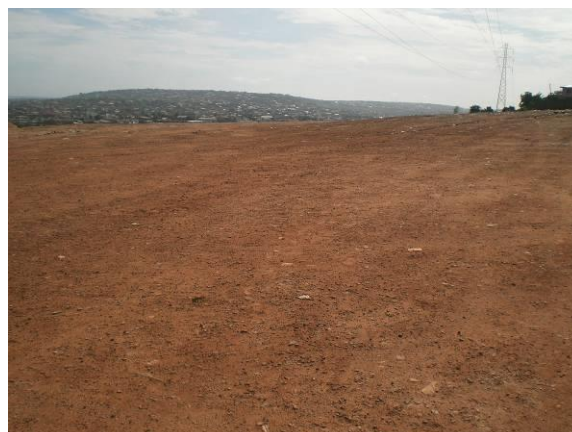
Plate 4: Final compacted surface after capping of the site
