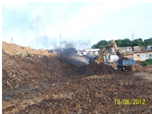
Plate 20: Formation of slopes and berms of Mallam No. 2
