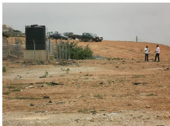
Plate 18: Attenuation tank in a protective fence on the completed capped surface
