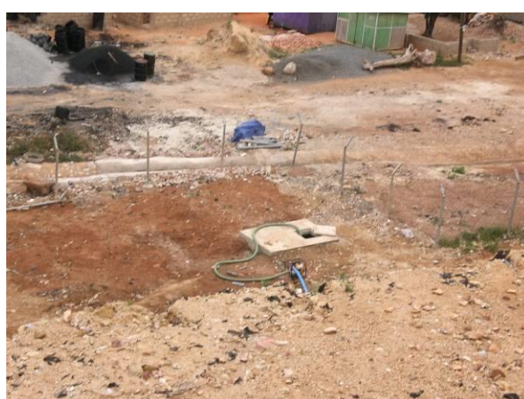
Plate 12: 10m 3 Concrete sump for leachate storage WC-SIRL system installed.
