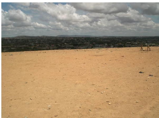
Plate 22: Final compacted surface of after placement of laterite layer
