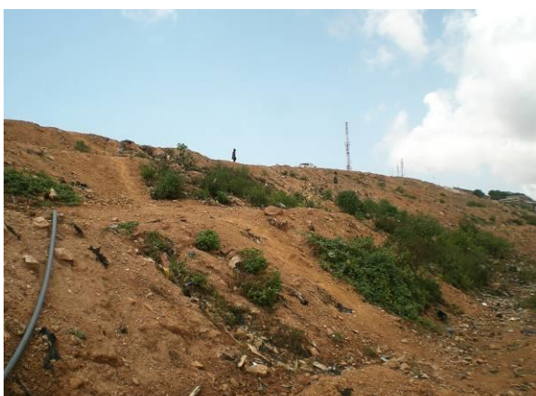
Plate 17: Completed slope surface with planted local shrubs
