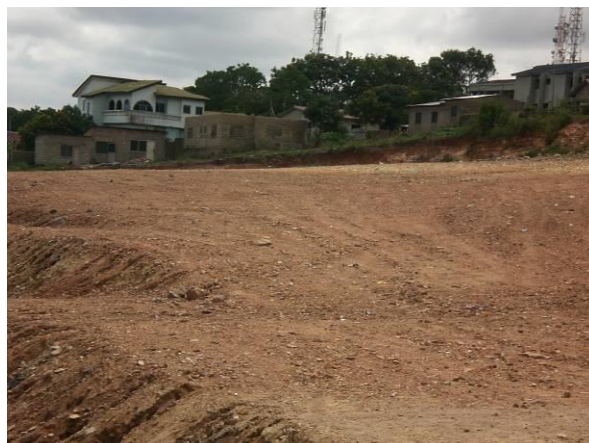
Plate 10: Final compacted surface after capping with laterite
