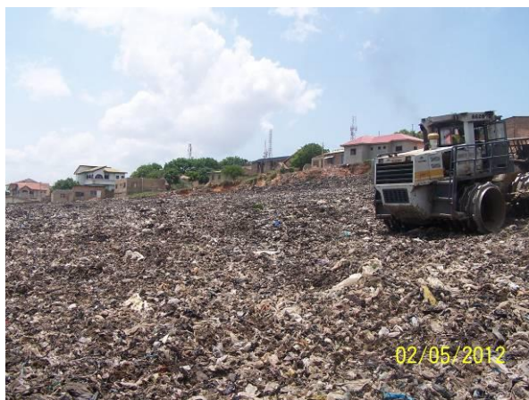
Plate 8: Levelling and compaction of refuse
