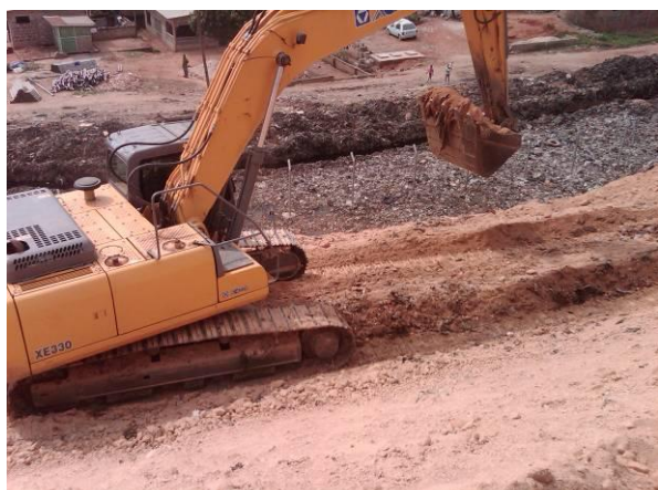
Plate 9: Grading to form slopes and berms
