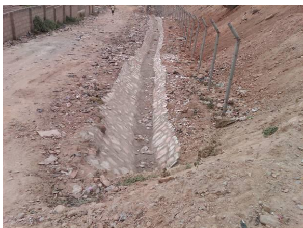
Plate 11: Stone pitched peripheral drain for conveyance of surface run-offs
