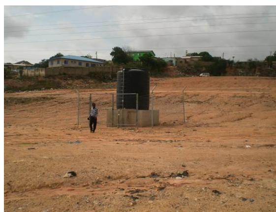
Plate 6: Attenuation tank in a protective fence. WC-SIRL system installed
