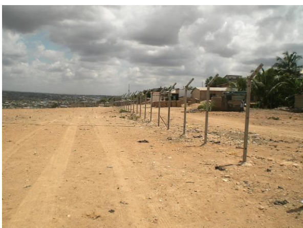
Plate 15: Final compacted surface of Mallam No.1 after placement of laterite layer
