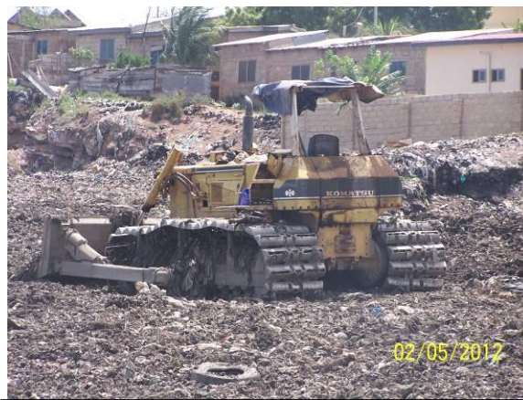
Plate 2: Levelling and compaction of refuse
