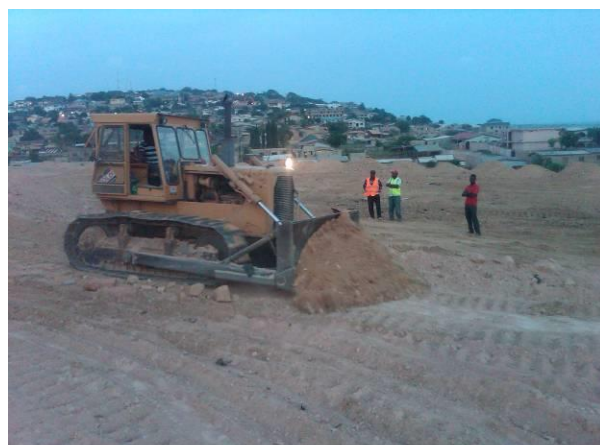
Plate 22: Placement and leveling of clay layer
