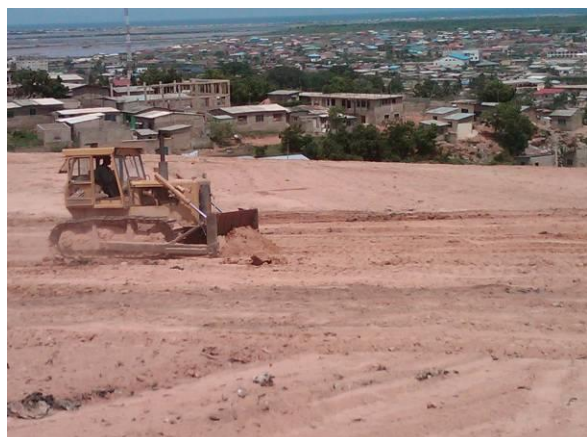
Plate 3: Placement and spreading of Clay – first layer
