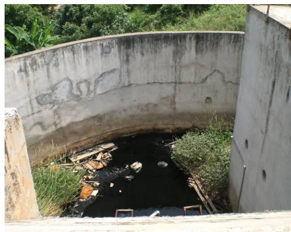
Plate 2-2: Collection well for leachate flowing from Oblogo No.1 dumpsite
