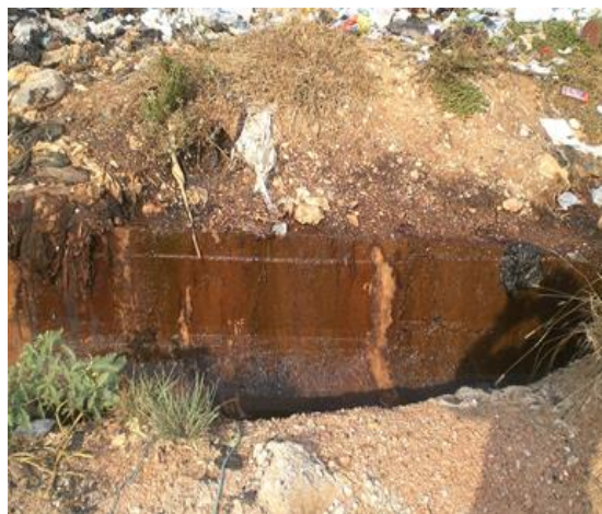
Plate 2-3: Flow of leachate from dumpsite into a u-drain
