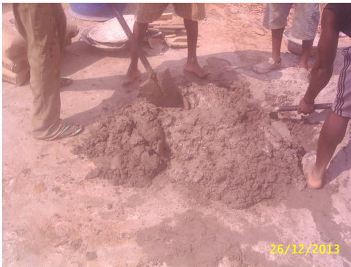
Preparation of mortar mix
