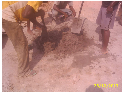
Preparation of mortar mix
