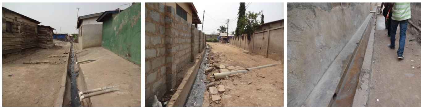
Plate 4.10: Greywater from house channelized into nearby open drains
