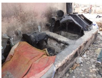
Plastic ventilators melted as a result of heat generated from the collection chamber
