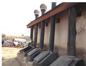
Plastic ventilators melted as a result of heat generated from the collection chamber
