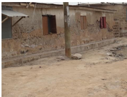
Plate 7.1: Cement block-made house walls showing signs of salt and water damage
