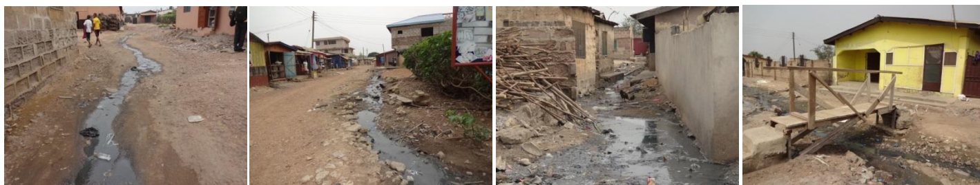
Plate 7.3: Evidence of poor drainage (lack of stormwater and sullage drains) situation in some parts of the community
