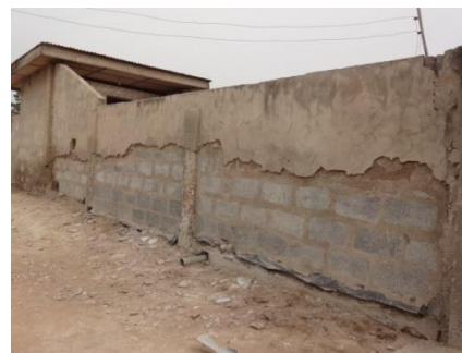
Plate 7.2: Rendering /plastering on fence wall wears off due to salt and water infiltration
