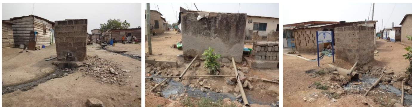
Plate 4.9: Bathroom wastewater disposal methods into earth drains
