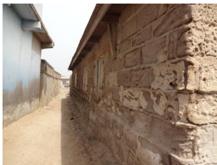
Plate 7.1: Cement block-made house walls showing signs of salt and water damage
