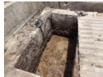
Exposed septic tank—has only a roofing sheet cover
