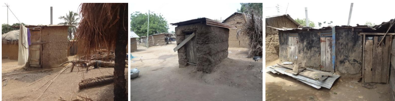
Plate 4.1: Examples of household toilets that are full and have been abandoned due to lack of desludging services
