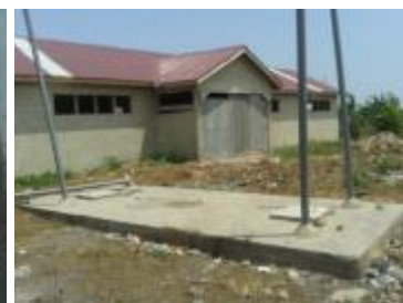
Septic tank with vent pipes
