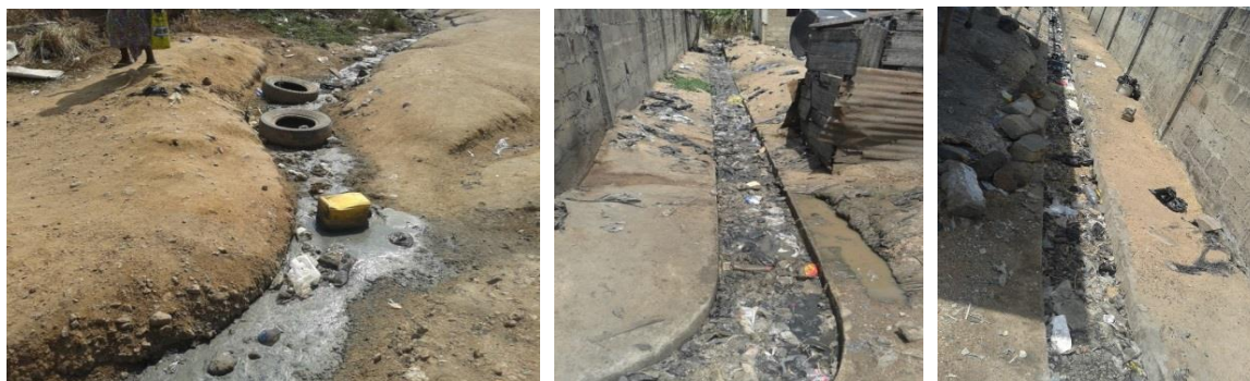
Plate 4.10: Disposal of sullage into earth drains and existing concrete drains filled with solid waste
