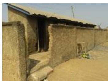
External view of the toilet facility showing damaged external wall
