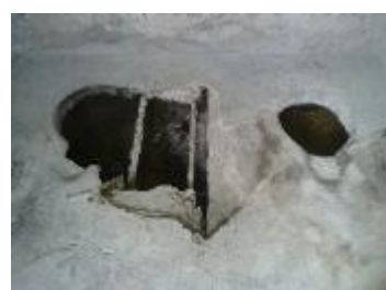
Damaged drops holes with reinforcement in concrete slab exposed
