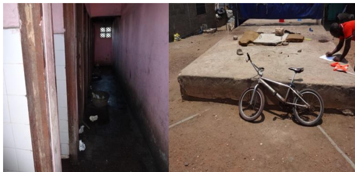
Plate 4.2: 12-Seater pour flush public toilet at Adedenkpo with soiled floor and broken septic tank slab.
