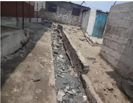
Plate 4.9: Tertiary drain within silted with solid waste
