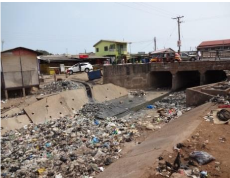
Plate 4.10: Major stormwater drain filled with solid waste
