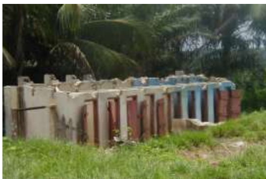
Plate 2.10: Demolished 20 seater public toilet.
