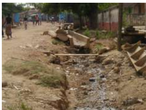
Plate 2.11: Storm drainage under construction by the community (with support from WSDB)
