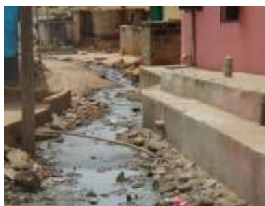
Plate 2.5 Shallow earth channel for sullage discharged from bathrooms
