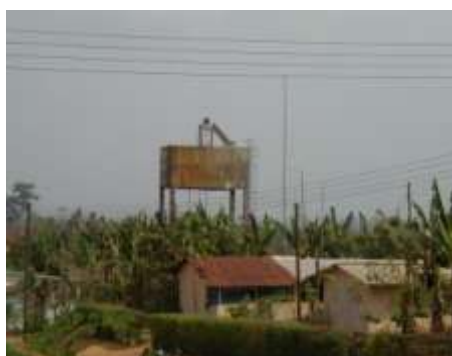
Plate 2.8: High level tank for water storage with an iron removal equipment
