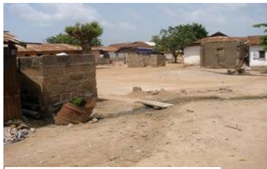
Plate 2.13 Shallow earth channel for sullage discharged from bathrooms
