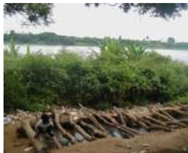
Plate 4: Latrine built with local materials without a superstructure close to the banks of Volta River, Asutsuare
