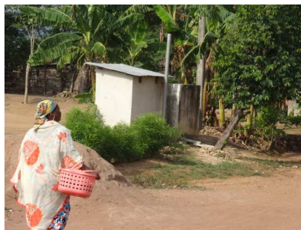
Plate 2.2: Household VIP in New Abirem with vent pipe extending from the base of the facility
