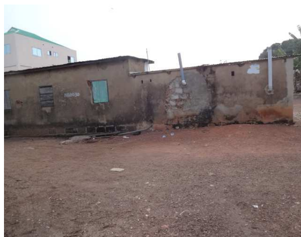
Plate 2.1: Household VIP in New Abirem with vent pipe close to the roof of the facility
