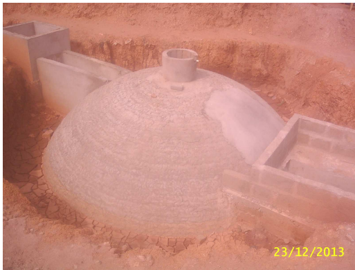
Bioreactor 1 – completed dome with inlet/outlet chambers
