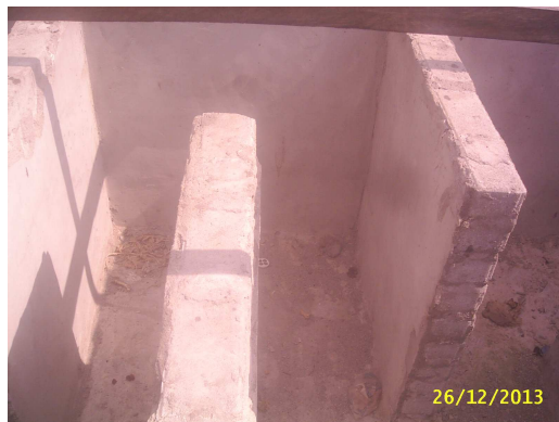
Solar water purification tank – showing baffles
