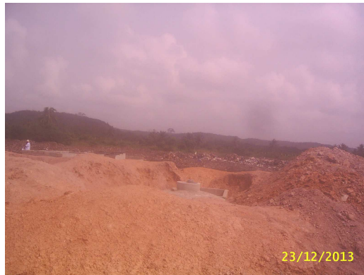
Bioreactor 2 – completed dome with inlet/outlet chambers
