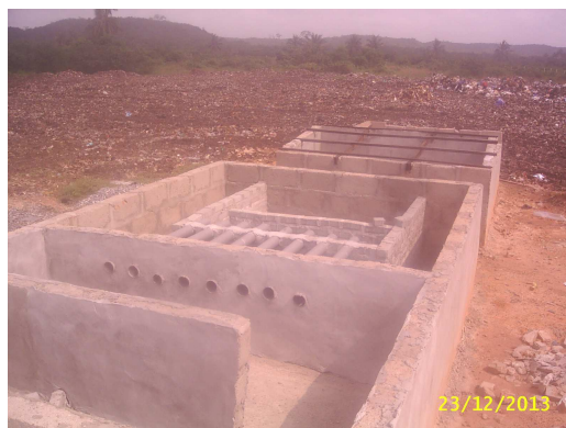
Hydro-Segregation tank under construction
