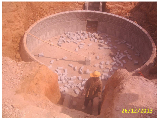
Bioreactor 4 – dome construction in progress
