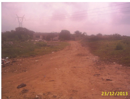
Poor access road to Project Site
