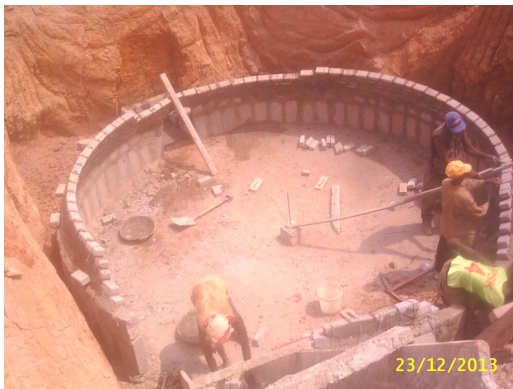
Bioreactor 3 – dome construction in progress
