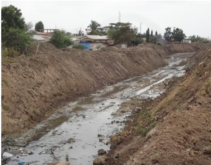
Plate 1: Unlined primary drainage
