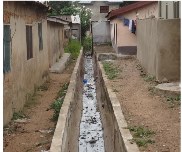
Plate 2: Lined concrete secondary drain
