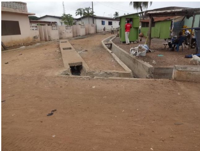
Plate 3: Road with side U drain
