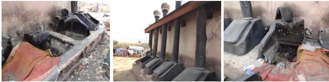
Plate 3.1: Melted vent pipes of the 10-seater Enviro-loo toilet
