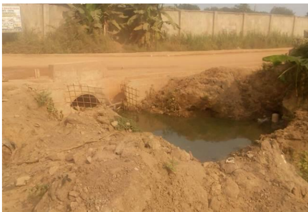
Plate 6.3: Culvert crossing on road
