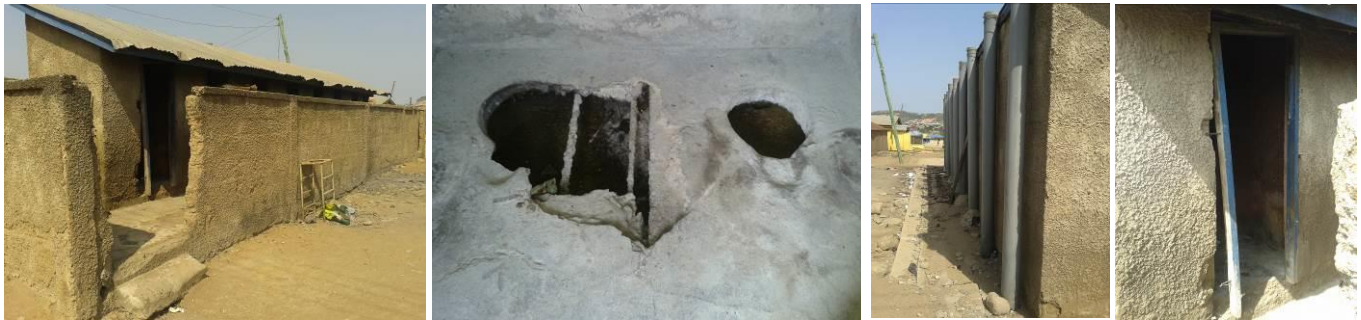
Plate 3.1: External and internal views of dilapidated 10-seater KVIP toilet at Galilea
