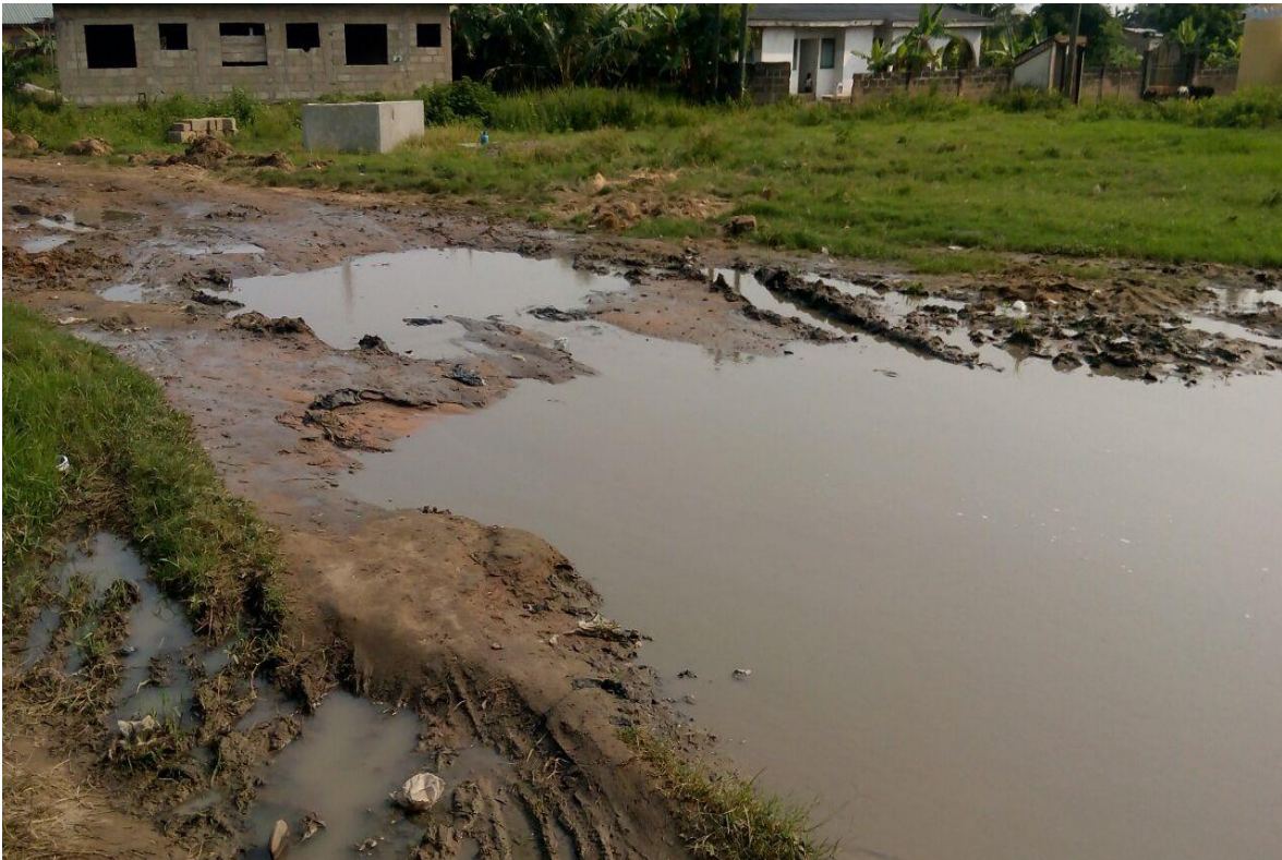
Plate 6.4 Ponding of road surfaces
