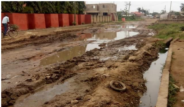
Plate 6.1: Un-engineered road with side drains
