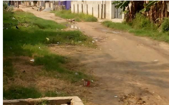
Plate 6.2: Un-engineered road without side drains
