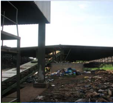
Plate3.11: Superstructure of the defunct Teshie Compost Plant showing the refuse conveyor belt.
