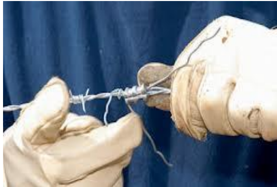
Repair/Replacement of damaged fence wires (Use protective gloves and pliers)
