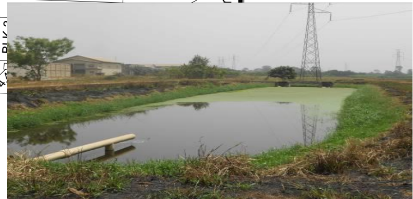
Plate : Additional anaerobic pond constructed to cater for institutional connections (Kumasi Polytechnic). Available land around ponds should be preserved against encroachment and for future expansions.
