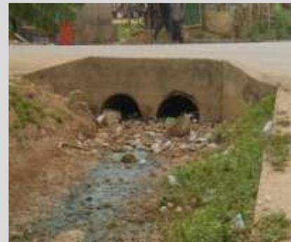
Plate 3.1: Circular culvert heavily silted with solid waste
