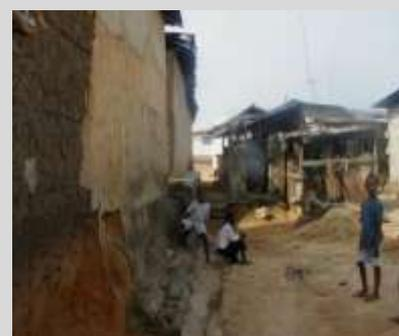
Plate 3.2: Extensive erosion which has exposed the foundation of a building
