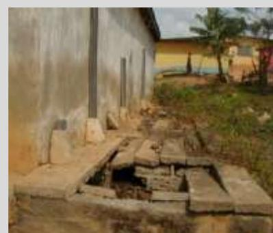
Plate 3.3: State of existing public latrine showing collapse of the holding tank
