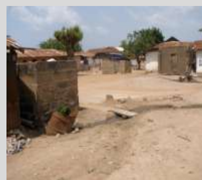
Plate 3.2: Wastewater from bathhouse disposed of through shallow earth channel into open space.
