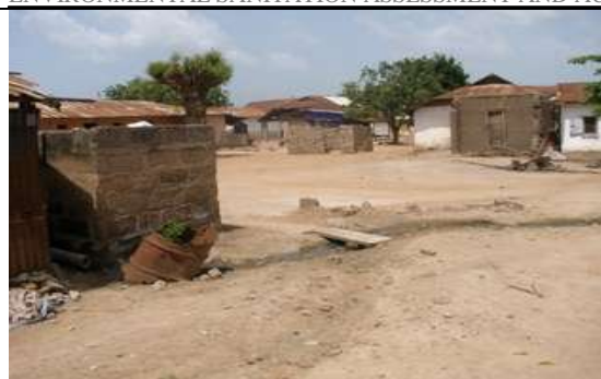
Plate 2.4 Shallow earth channel for sullage discharged from bathrooms
