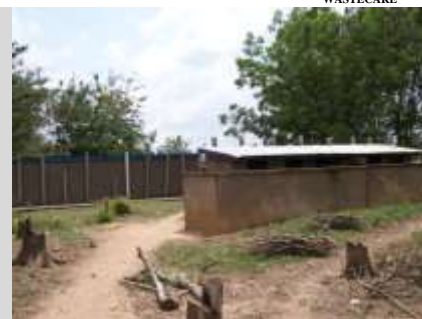
Plate 3.4: The DA primary and JSS 8-seater KVIP toilet facility provided by CWSA.
