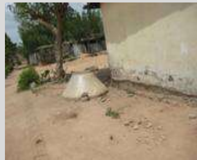
Plate 3.1: Exposed foundation due erosion.
