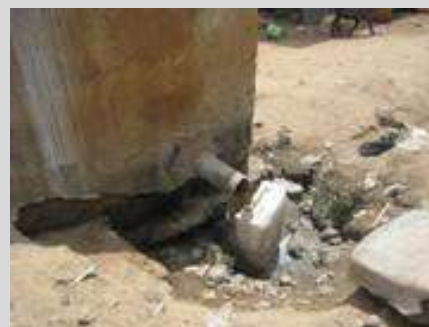
Plate 3.2: Wastewater from bathhouse disposed of into earth soakage pit.
